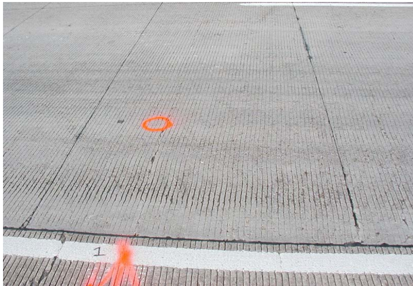
Figure 6.9 Test section at SH 225 with sawcut
