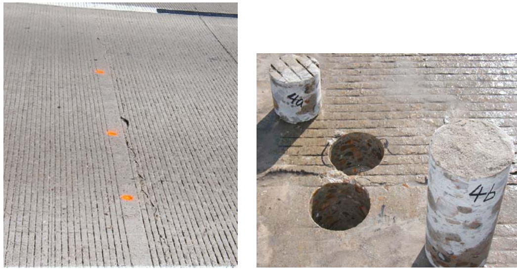
Figure 6.15 Crack #4 and concrete cores
