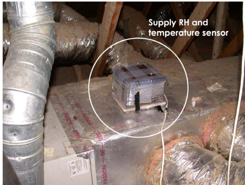
*Figure 4.11 Supply temperature / relative humidity sensor with insulation*
