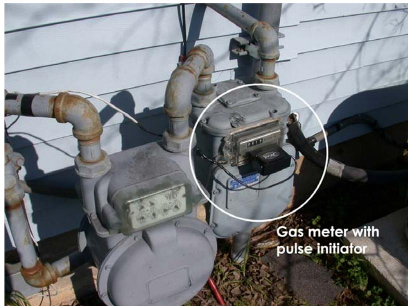
*Figure 4.14 Gas meter with pulse initiator*
