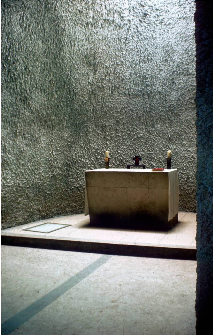
Figure 14: Interior: Northwest side altar. (Archive Colour Slides Ltd., 1984, Slide 10 L 24,062)
