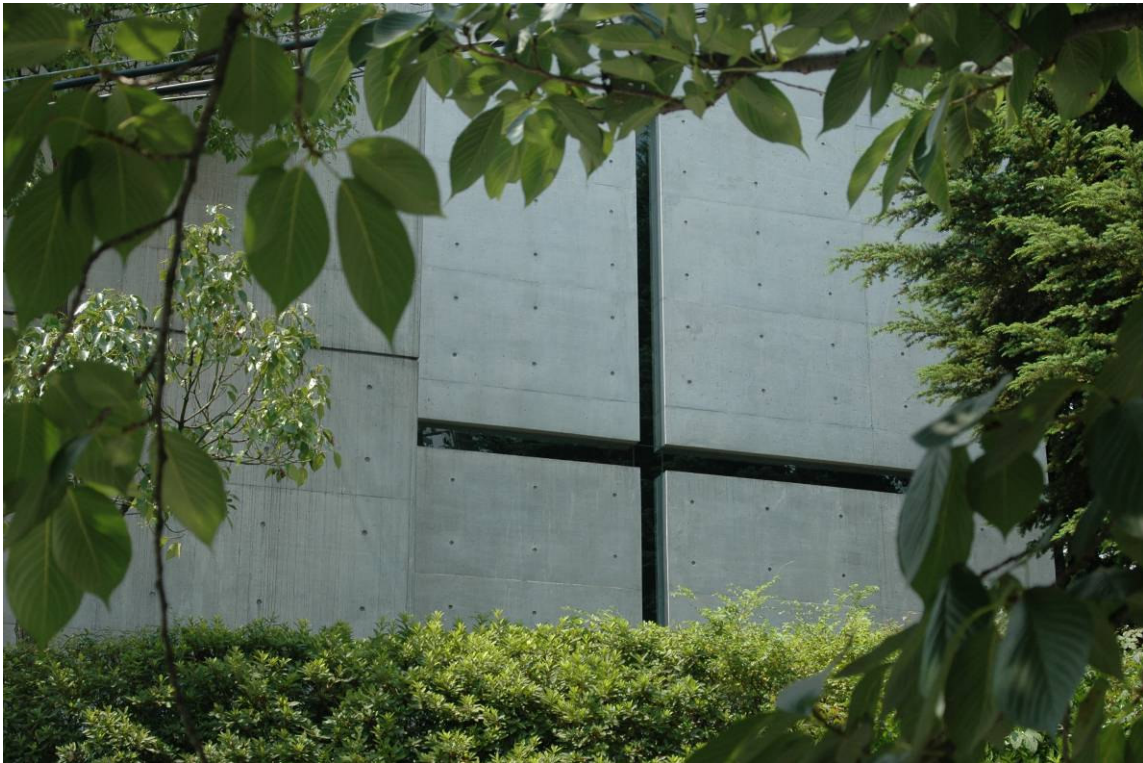
Figure 40: Exterior view of the Church of the Light showing the cross cut in the concrete wall.
