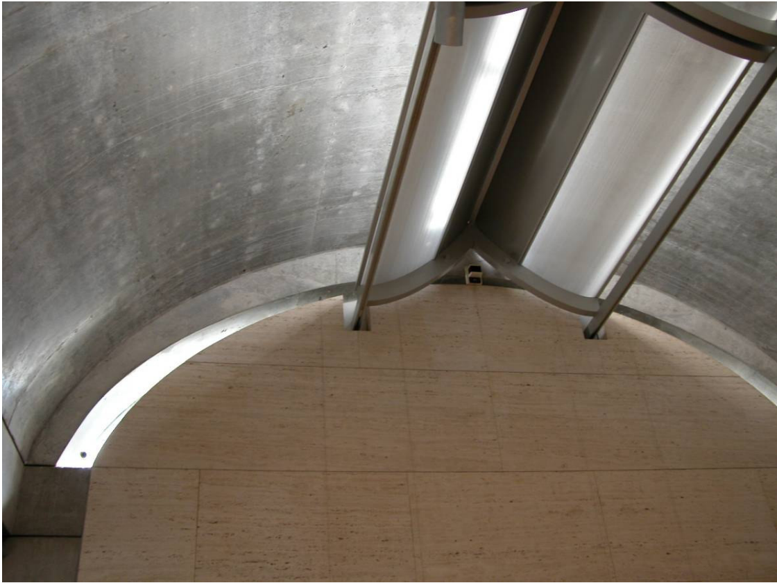
Figure 35: The effect of light on the irregularities of two similar surfaces. (Photo courtesy of M.M.H. Alnuaimi, 2005)
