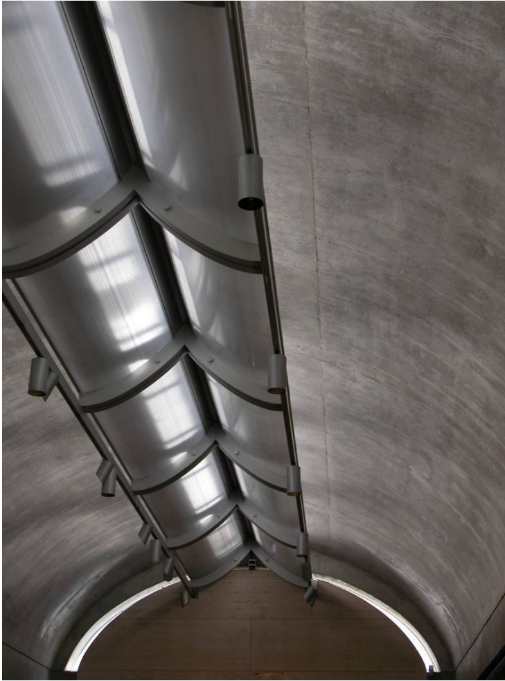
Figure 31: The penetration of the spatial envelope towards the gable end. (Photo courtesy of M.M.H. Alnuaimi, 2005)
