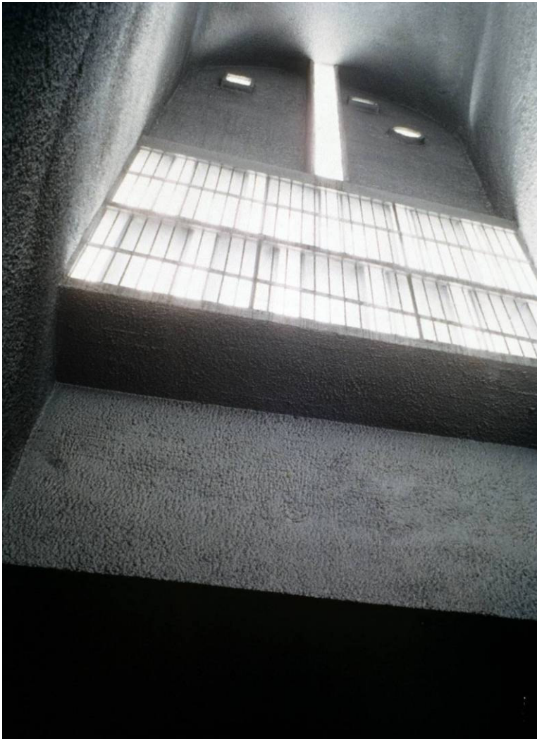
Figure 13: View up into main tower from the south. (Archive Colour Slides Ltd., 1984, Slide 10 L 24,064)
