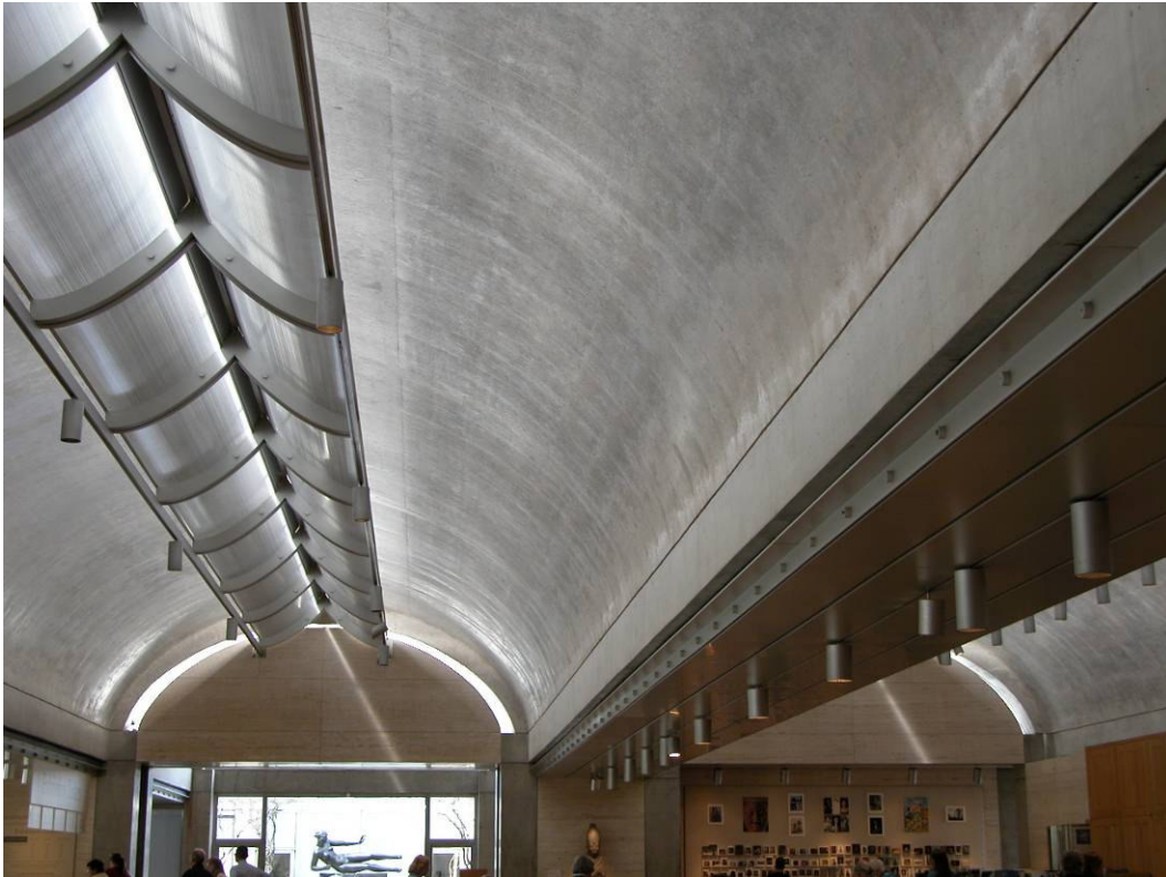
Figure 27: Interior view showing the even distribution of light from the daylight fixture. (Photo courtesy of M.M.H. Alnuaimi, 2005)
