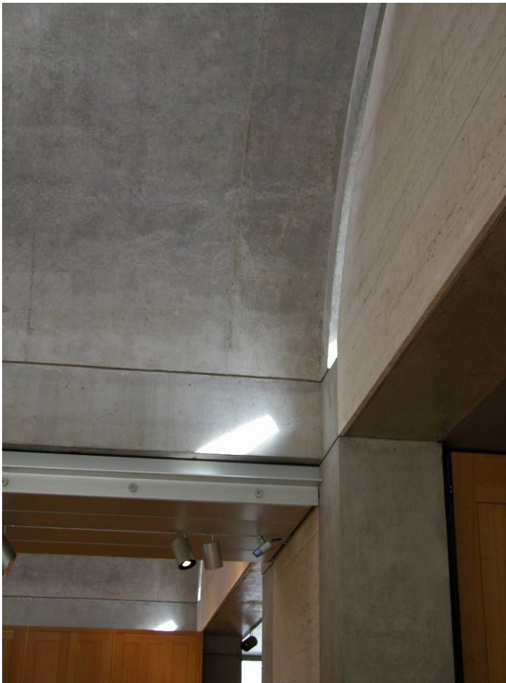
Figure 33: The 3' expansion joint on the south end of the spatial envelope. (Photo courtesy of M.M.H. Alnuaimi, 2005)
