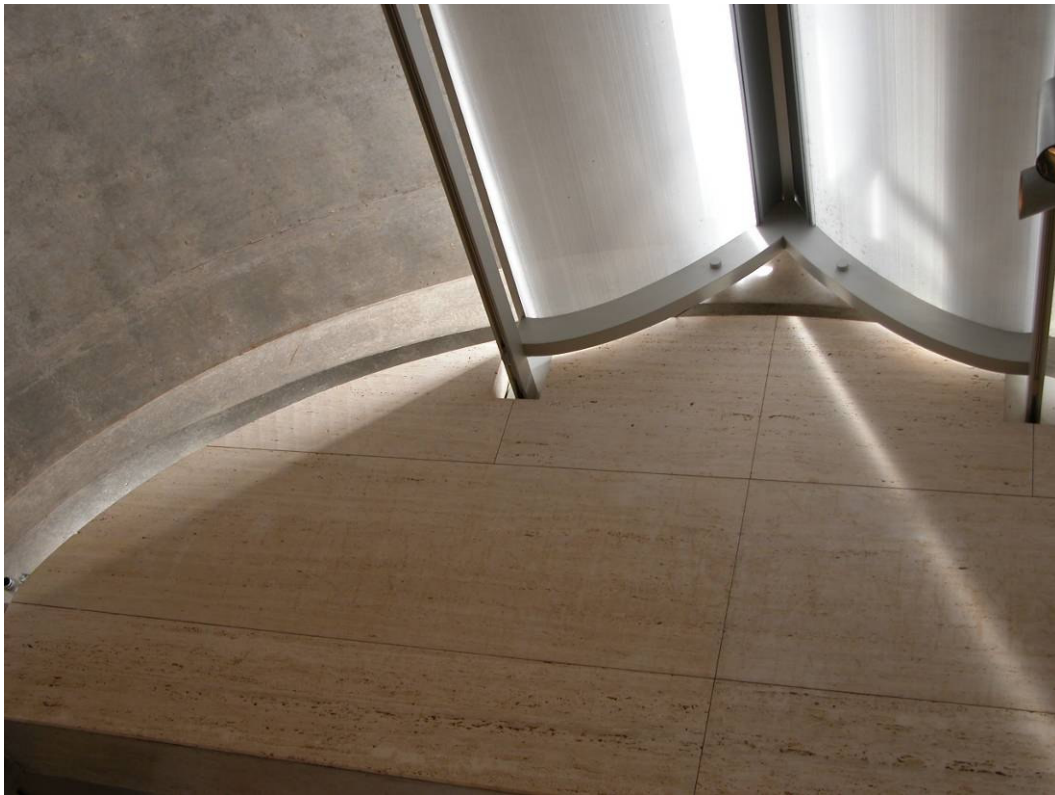
Figure 38: Effect of light as it enters from the gap between the cycloid shell and gable end of the circle. (Photo courtesy of M.M.H. Alnuaimi, 2005)
