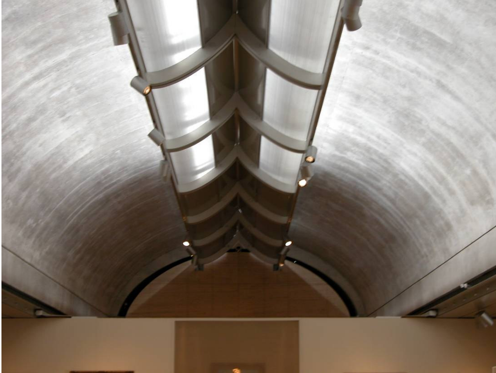
Figure 25: Interior view of the ceiling with the daylight fixture. (Photo courtesy of M.M.H. Alnuaimi, 2005)
