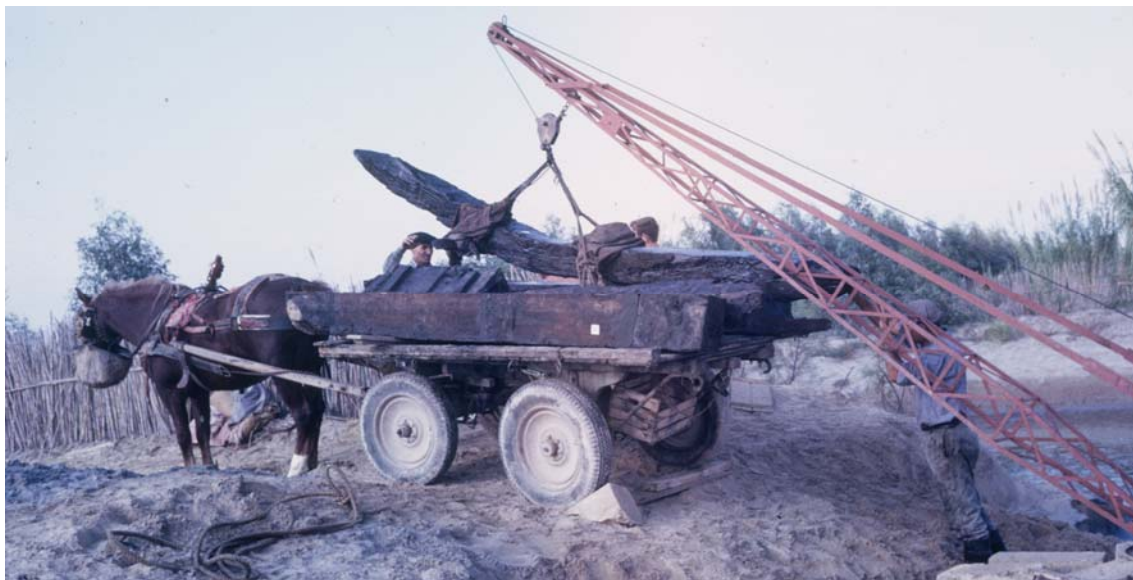
Fig. 3.3 A horse-drawn crane and wagon moving timbers from the site to Francesco Spatola's irrigation tank (courtesy INA Archives).
