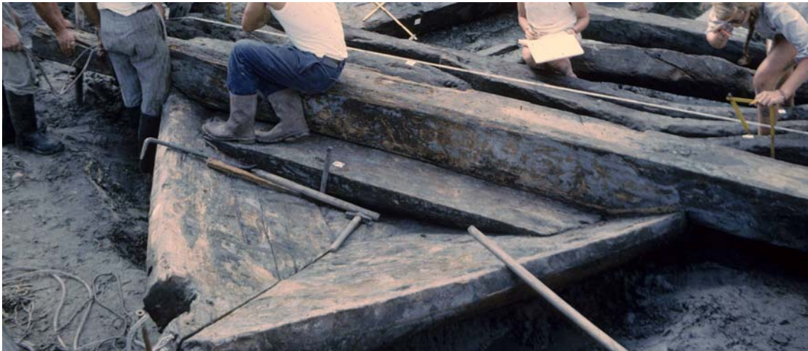
Fig. 6.12 Supporting transverse timbers are revealed during the disassembly of the ramp (Photograph: Johann Reinhard).
