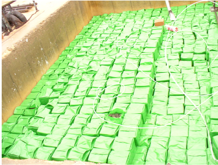
Figure 20. Foamglas(R) PFS installation in a containment dike
