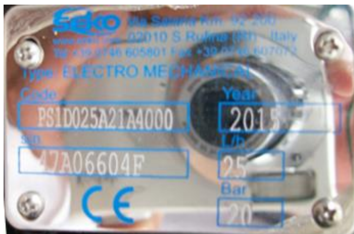
Figure 5-7: License plate of the pumps.
