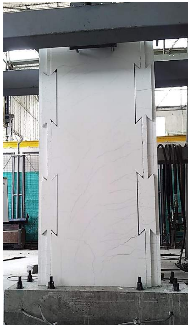
b) Damage state DS_2
