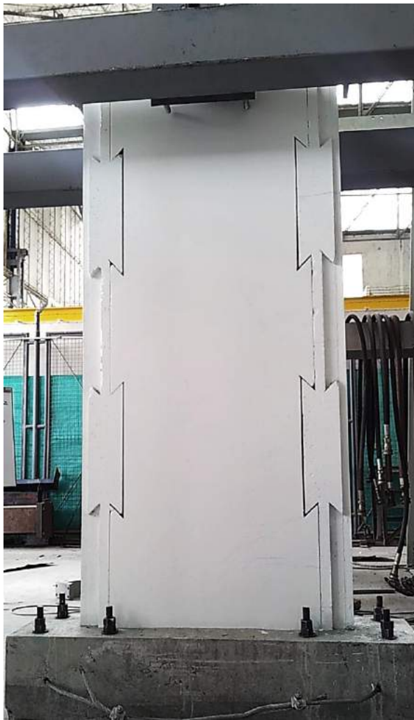
a) Damage state DS_1
