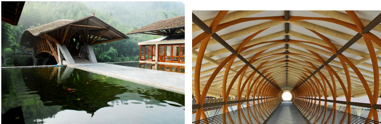
Figure 1.1: Two constructions by Simón Vélez, Architect. Guadua culms were used as the construction structural material. (Left) “Puente en la China” (Bridge in china).[Vél]. (Right) , 2009 Simón Vélez, Principal Prince Claus Award in the Netherlands [Kra11].
