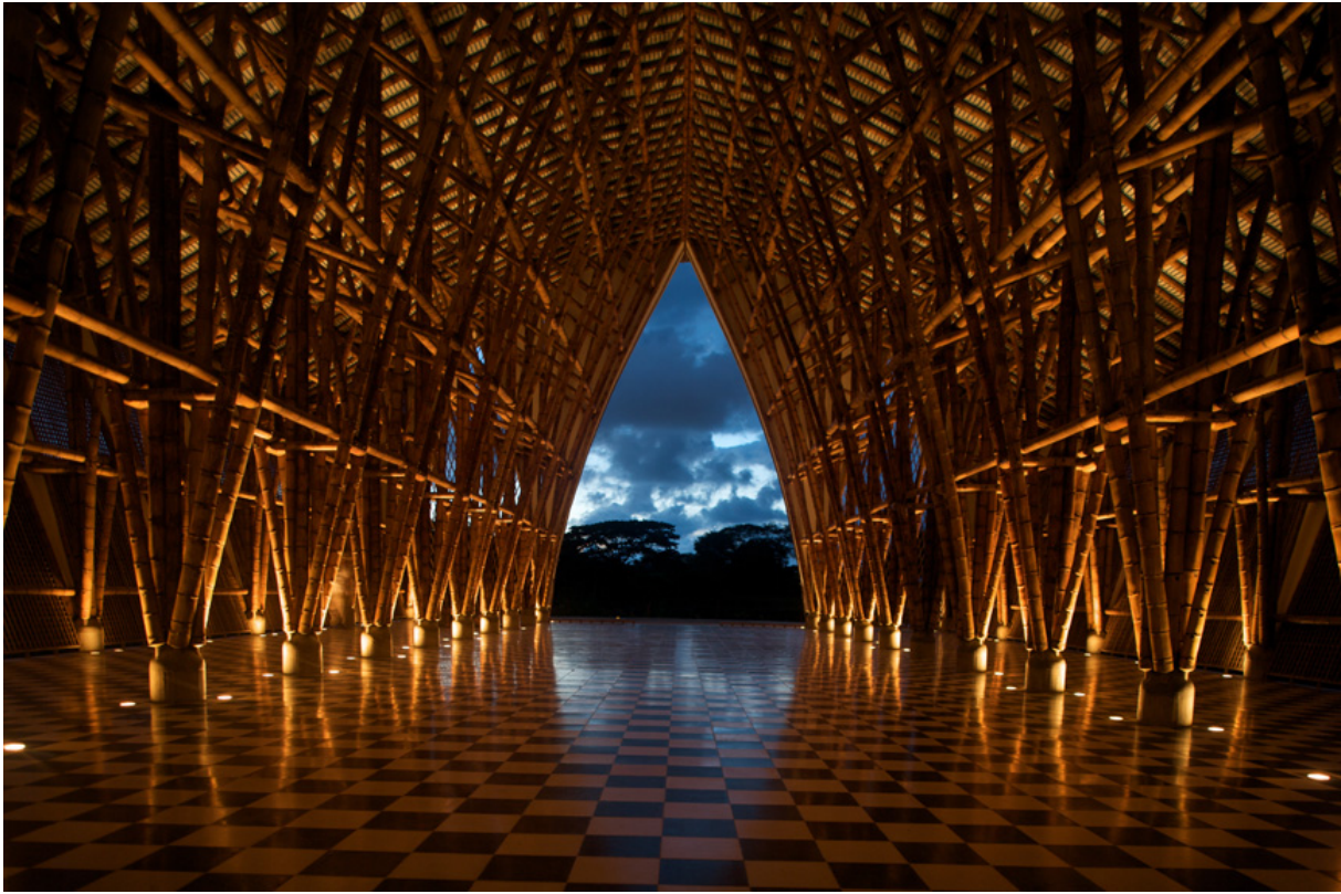
“Iglesia sin religión, interior” (Cultless church), Simón Vélez, Architect. Guadua culms were used as the construction structural material. [Vél]
