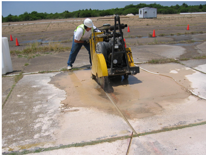
Fig. 32. Sensor bar installation: Saw tooth cutting the slot in the road
