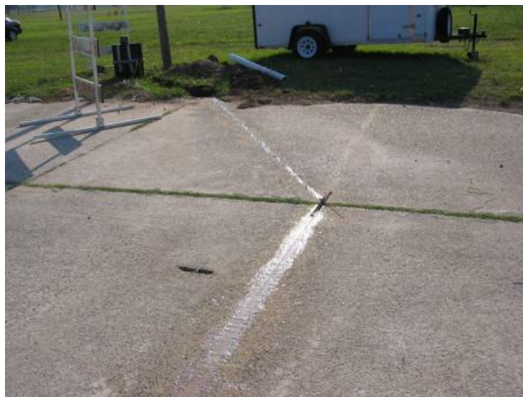
Fig. 34. Sensor bar installation: Final appearance after the epoxy and sealant have dried
