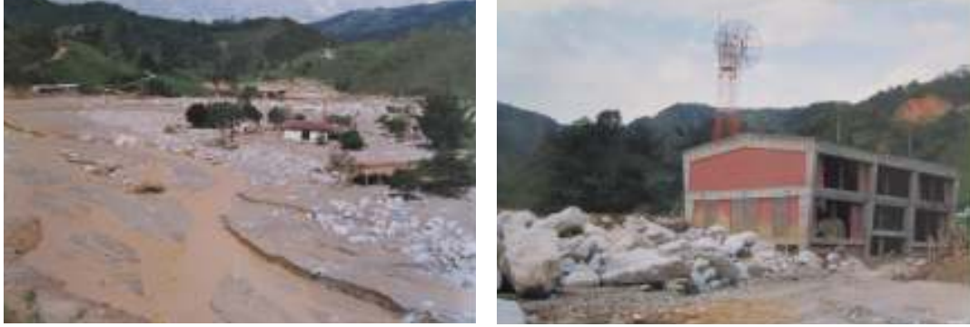
Figure 1.8 Landslides material removed from the upper catchment slopes was later carried away by runoff producing torrential floods that destroyed 27 houses (left picture) and severe damaged to the Calderas Hydroelectric Plant of ISAGEN (right picture) (Taken from Mejía & Velásquez, 1991).
