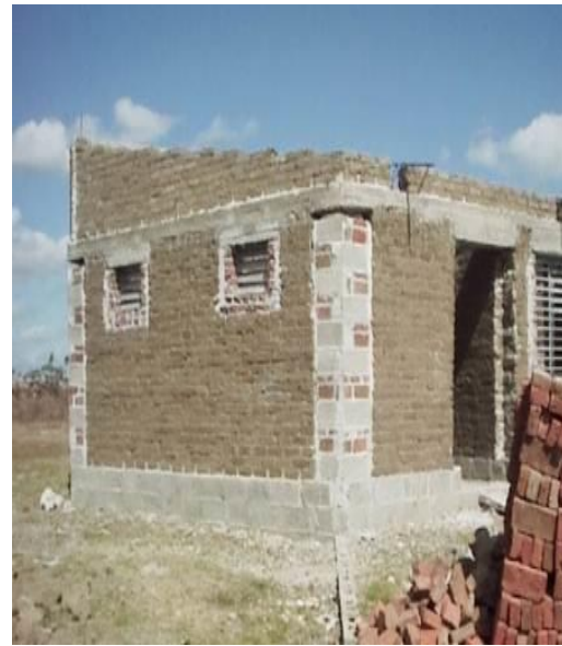
Figure 3: Hollow blocks foot cords
