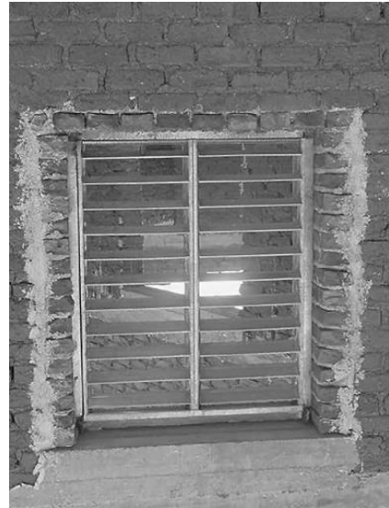
Figure 7: Adobe wall, mortar number three and fired bricks
