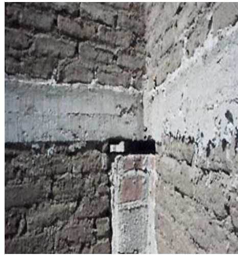
Figure 11: Pillar plural o singular 10 cm shorter than the wall
