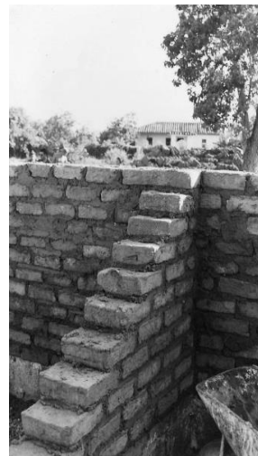
Figure 13: Solution for the lower lintel
