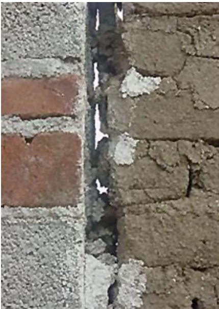
Figure 9: Only pillars supporting the collar beam
