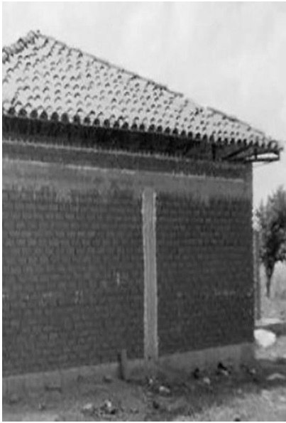
Figure 5: Wall with an intermediate pillar
