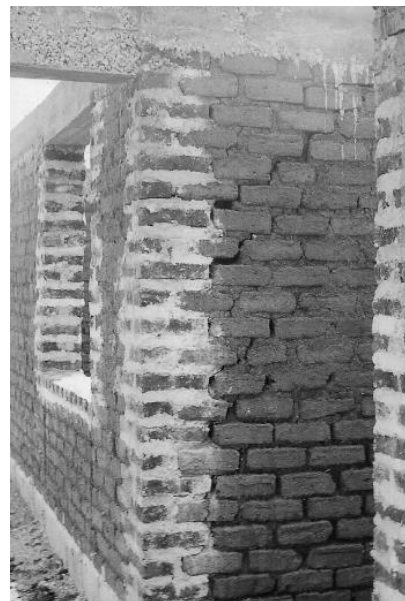
Figure 8: Wall and pillar supporting together the collar beam
