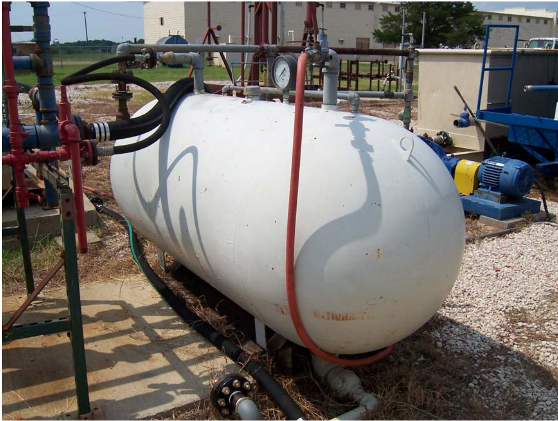
Fig. 4.5 – Pressure equalization vessel.
