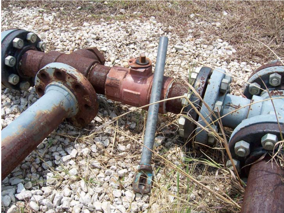
Fig. 4.7 – Backpressure control valve.
