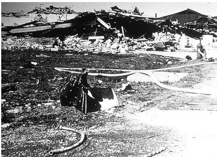
Figure 4 Plant laboratory after EO vapor cloud explosion-300 feet away
