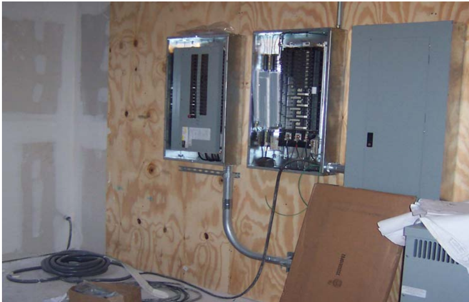
Figure 15. Electrical Panel Installation for Project C
