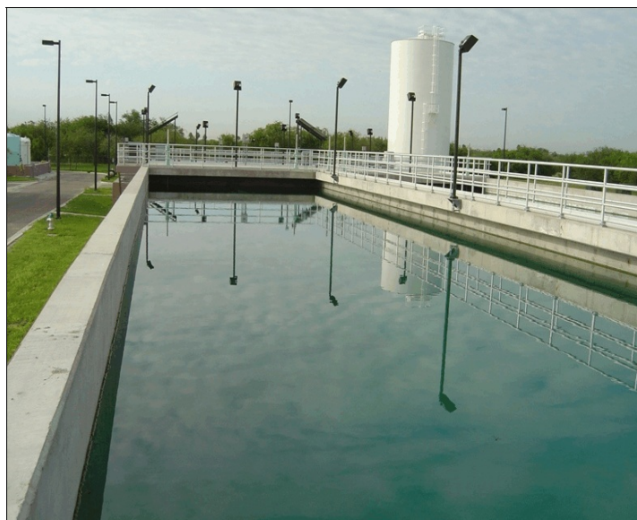
Figure 6. Sedimentation basins at McAllen Northwest facility
