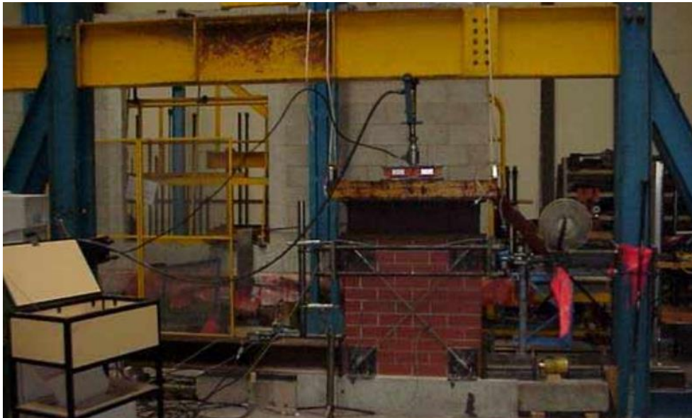
Imagen 3.3.1-1 Ensayo del murete. Fuente: CHUANG, S., ZHUGE, Y y MCBEAN, P. Seismic retrofitting of unreinforced masonry walls by cable system . Vancouver, B.C., Canadá: s.n., 2004. 13th. Word Conference on Earthquake Engineering. Paper No. 3228.
