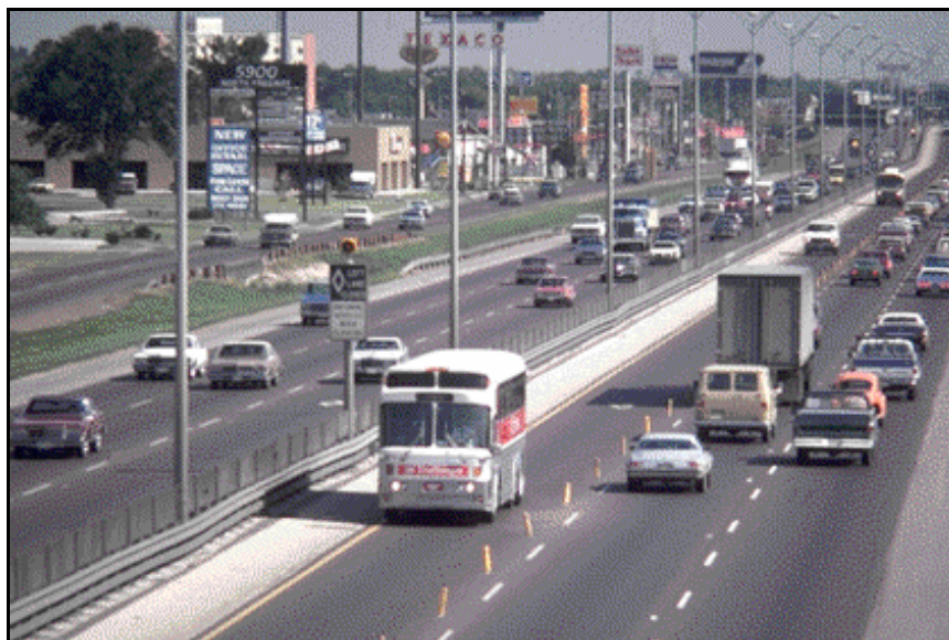
Figure 2.8. I-45 contraflow lane (Courtesy of TTI)
