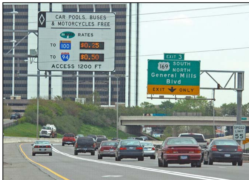
Figure 2.5. MnPASS toll rate sign (Courtesy of Lee Munnich)
