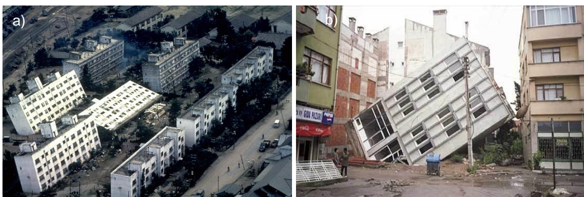
Fig. 2. a) Overturning failures in residential complex in 1964 Niigata earthquake, and b) Liquefaction-induced settlement due to loss of bearing capacity in 1999 Kocaeli earthquake (after NISEE 2016).
