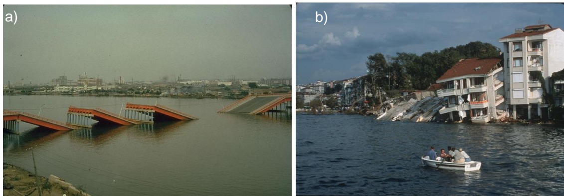
Fig. 3. a) Lateral spreading causing bridge spans to fall off from its supports during the 1964 Niigata earthquake, and b) Lateral spreading of waterfront properties during the 1999 Kocaeli earthquake (after NISEE 2016).
