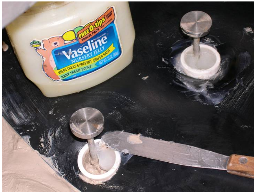
Fig. 4.32. Sealing the rubber cover holes.
