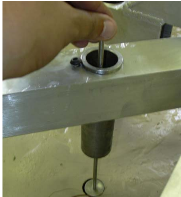
Fig. 4.24. Installing the extension stems with pedestals.
