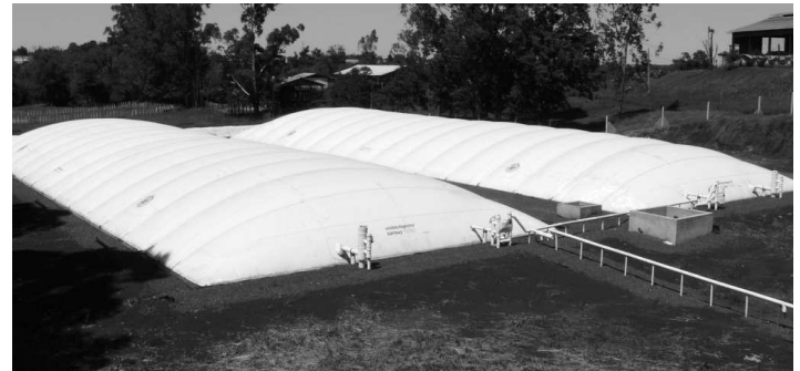
Fig. 3: Biodigesters at the San Bernardo Farm of Naranjal, Alto Paraná (Foto: Pulfer)
