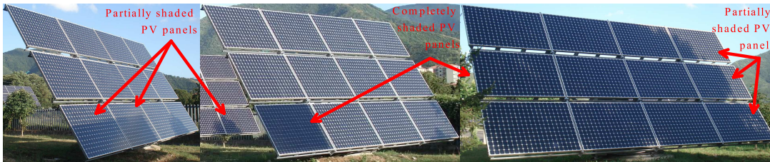
Figure 1-2.: Shading profiles affecting PV systems.
