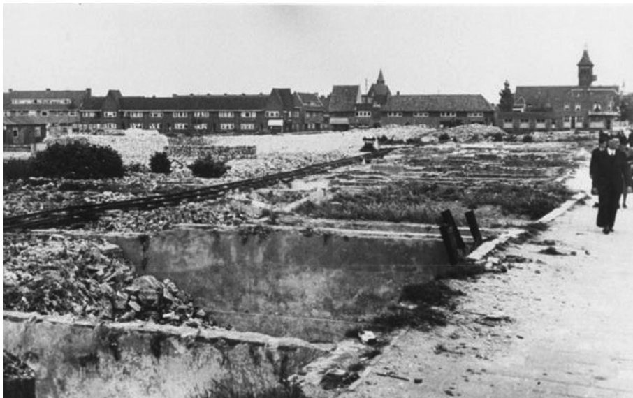
Figure 8b. The western part of the neighbourhood is completely demolished. The eastern part is untouched, which is visible in the background of the picture. Photography: A. Magrijn-Hooiveld (1943).
