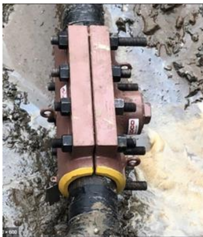
Fuente: Split Sleeve Installation for pipeline repairs by PLIDCO.
