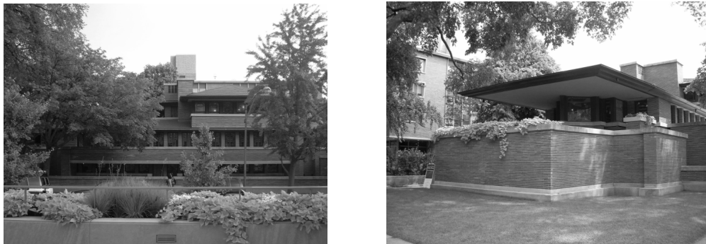
Fig.4.10 – Horizontality in the Robie House. Left: The horizontal planes on the lower floors change to piers and larger opening on the top floors. Right: The hipped roof projects beyond the confines of the Robie House. (author)
