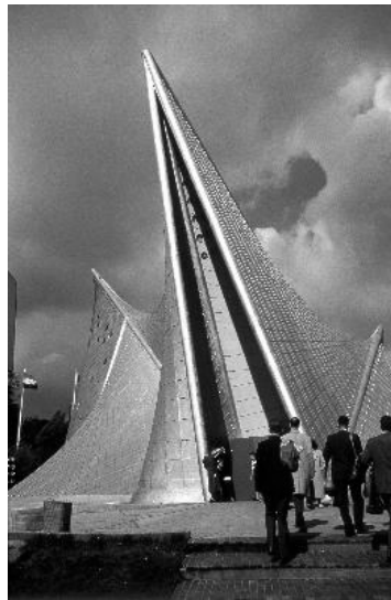
Fig.6.2 - Philips Pavilion, 1958, World's Fair, Brussels. From John Donat/ RIBA Library Photographs Collection/ FLC/ADAGP, Paris and DACS, London 2008. ( www.architecture.com ).
