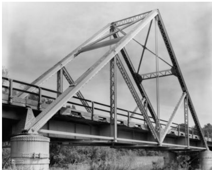
Figure 1.1 Configuration of Waddell "A" Truss Bridge.
