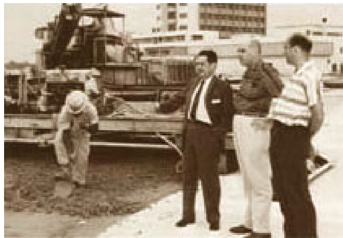
Figure 1.6 Pavement Construction at Miami International Airport.
