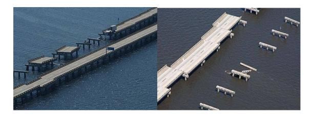
Figure 4.2: I-10 Bridge destroyed by Hurricane Ivan across Escambia Bay in Sep, 2004
