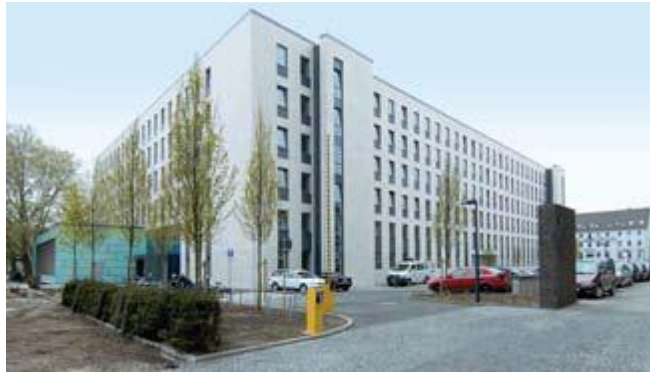
Figure 3.20 Neues Regionshaus Hannover Building
