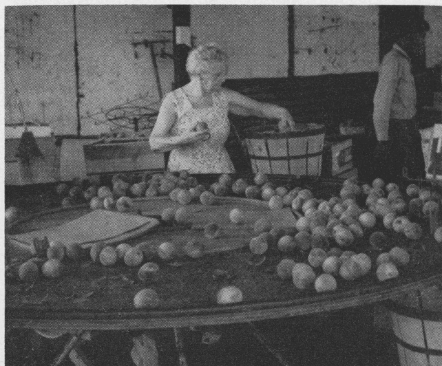
Figure 8. Revolving tables are common in many new packinghouses.
