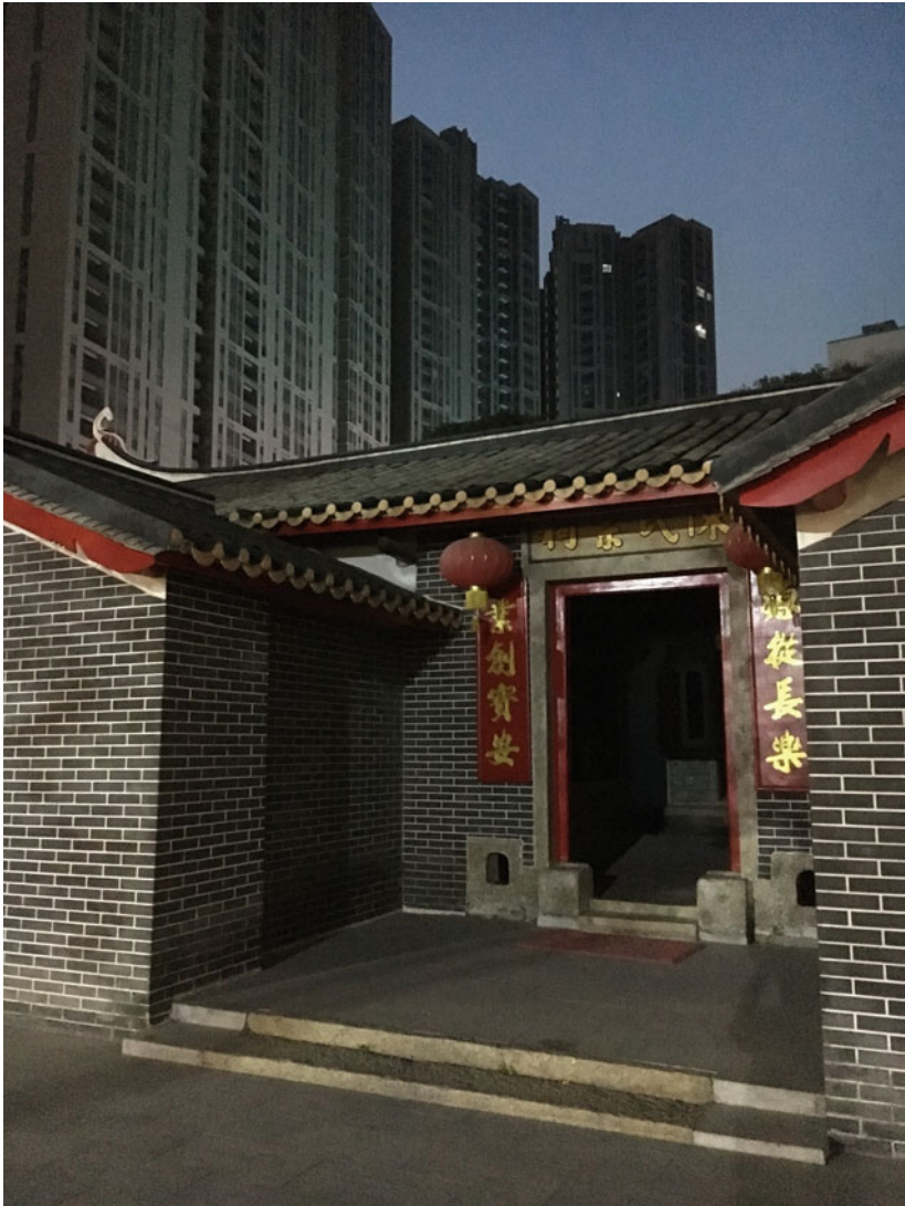
Fig. 2.1 Renovated lineage temple surrounded by high-rise buildings (Photo by author)
