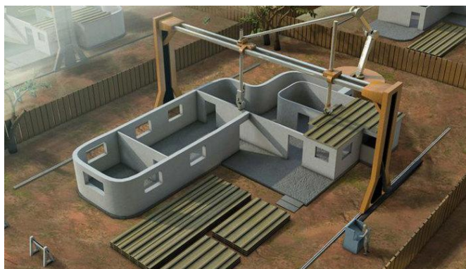
Figure 4. Contour Crafting develops 3D printing technology pioneered by Berokh Khoshnevis at the University of Southern California (2020)
