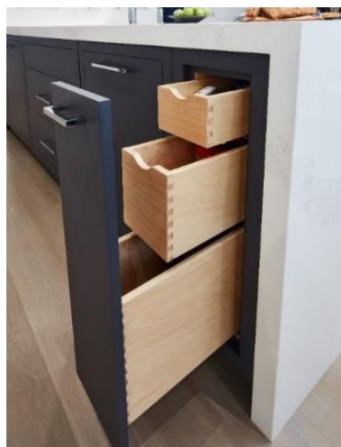
Figure 104 - One drawer and two roll out shelves nested in a box family
