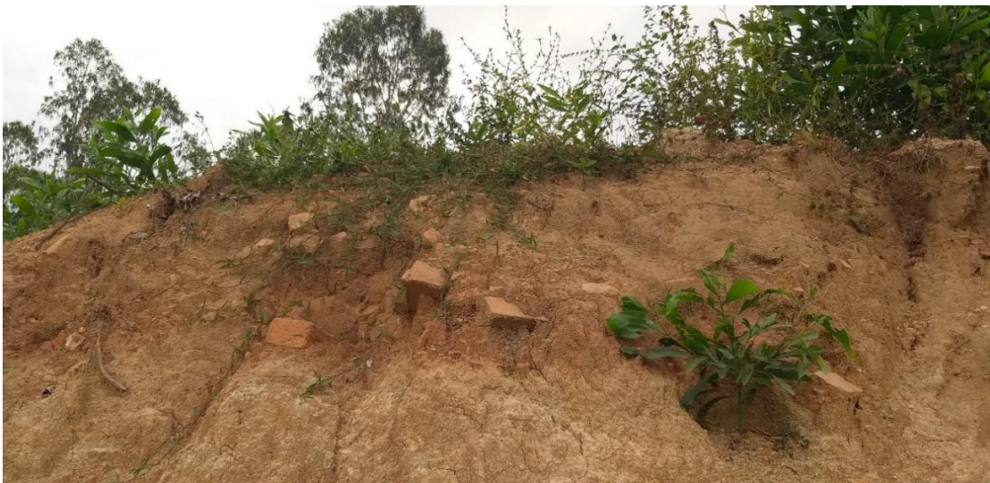
Fig 2. 49: Bricks scattered on the ground in Go Gạch Tam Xuân 1
