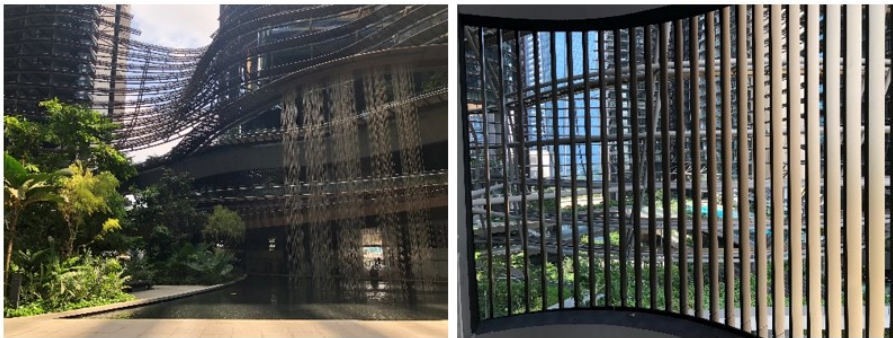
Figure 9. Louvers, waterscape and permeable external walls of Marina One
