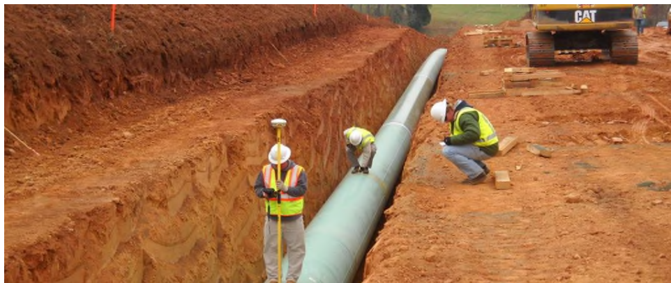
Fig. 1. Laying of linear objects (gas pipeline, power transmission lines, etc.).
