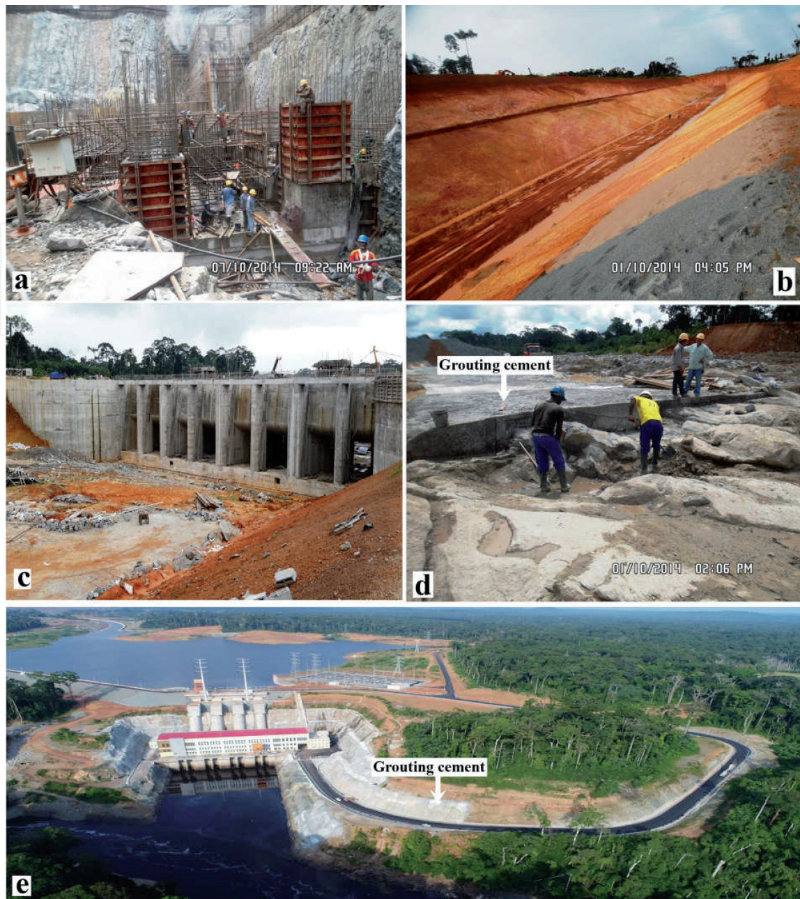
Figure 8. (a–c) Display different usages of Ntem formations and quaternary soil deposits; (d and e) amendment of Ntem formations and slope formed by quaternary soil deposits with grouting cement.
