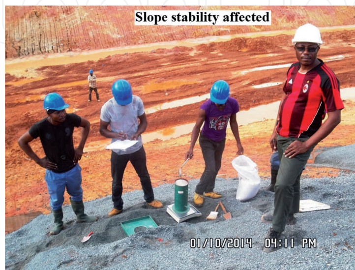
Figure 5. Slope stability affected by raining water.
