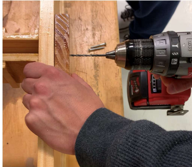
Figure 22: Drilling pilot holes for side supports
