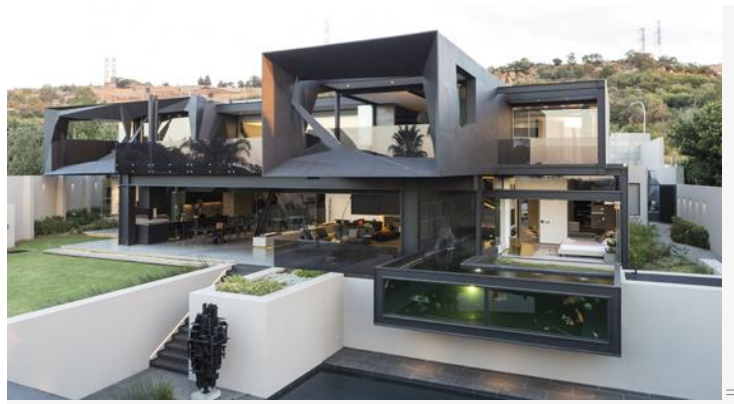
Fig.2: Nico van der Meulen Architects, integration of the smart-home technology (archello,2017), (Source: M Square Lifestyle Design).
