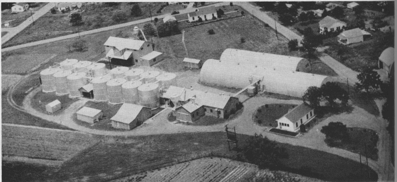
Figure 2. Processing and storage facilities of a cotton planting seed organization. Courtesy of Texas Planting Seed Association, Bryan, Texas.
