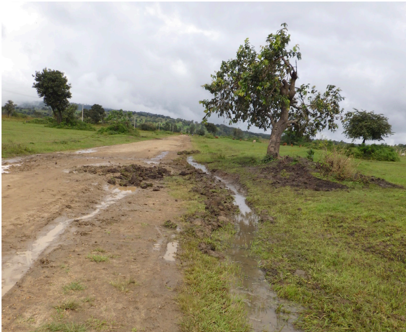
Figure 9. Mud Excavated from the Drainage onto the Main Surface
