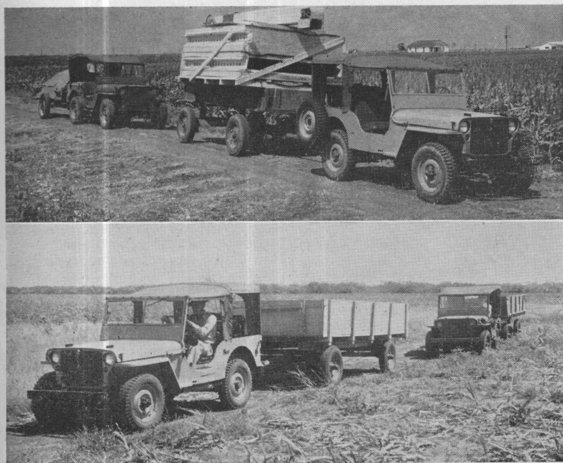
Fig. 12. Jeeps pulling trailers. Top—The Universal jeep (in front) pulling a four-wheel trailer loaded with a knocked-down grain dryer, and the military jeep pulling a two-wheel trailer loaded with miscellaneous equipment. Bottom—Both jeeps pulling four-wheel trailers loaded with milo from the field.
