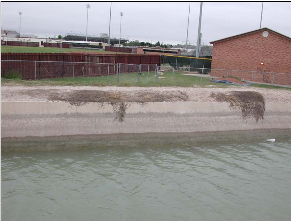
Figure 5c. Site 4 – Photograph showing the dead grass along the canal and that the canal segment is in good condition
