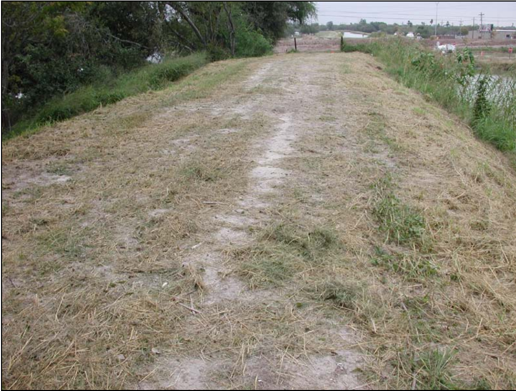
Figure 2d. Photograph showing dirt road on canal embankment at Site 1.
