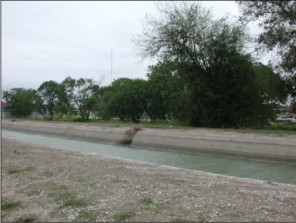
Figure 3c. Site 2 – thick vegetation along the canal.
