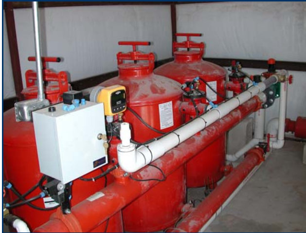
Figure 5. Sand media filters are preferred when silt and fine sand are problems with the irrigation water. System controllers (right panel) are programmed to set the length of time and time of day and/or day of week fields are to be irrigated.
