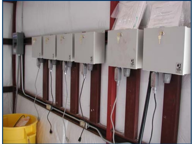
Figure 5. Sand media filters are preferred when silt and fine sand are problems with the irrigation water. System controllers (right panel) are programmed to set the length of time and time of day and/or day of week fields are to be irrigated.
