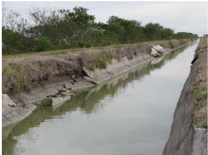
Figure 1. Main 'J' Canal
