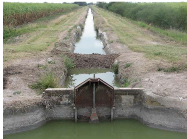
Figure 4. Lateral gate & earthen dam downstream
