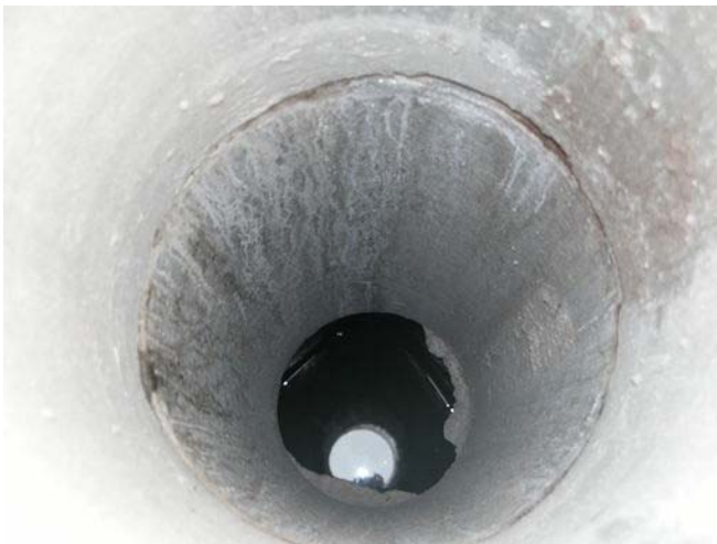
Figure 5. Inside view of a 12 inch standpipe and box structure.
