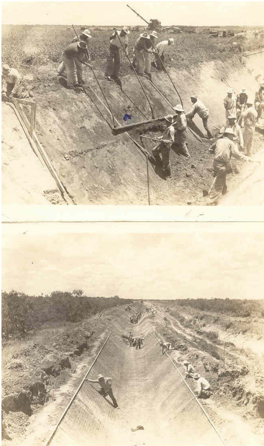
EXHIBIT C3. Construction of the Main J Canal to Raymondville, 1930 (Harding Collection).
