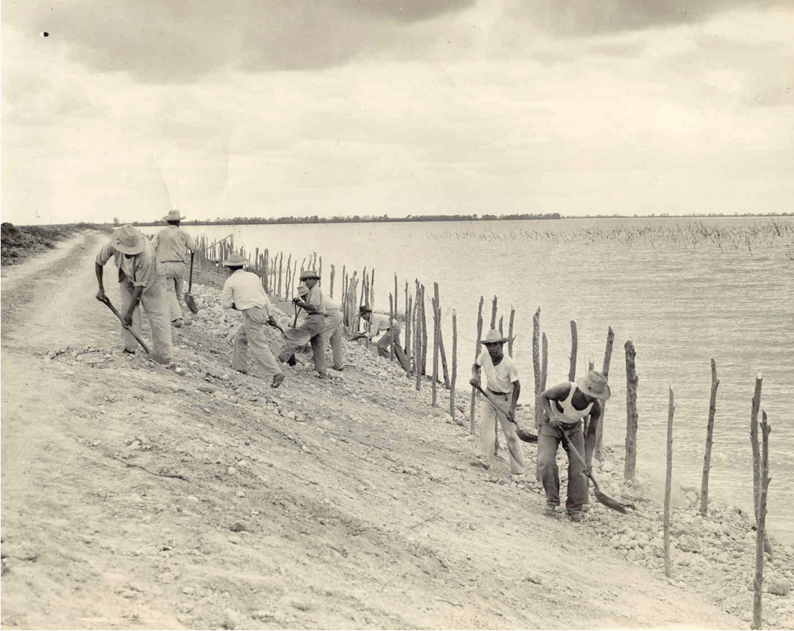
EXHIBIT C4. Construction of Erosion Control Measures on the Shores of Delta Lake, 1935 (Harding Collection).
