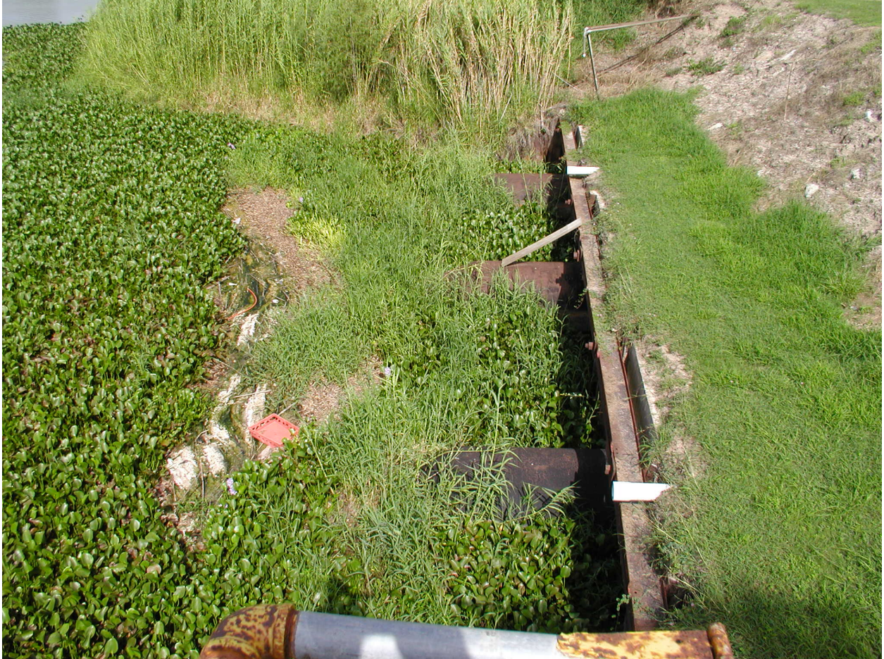
EXHIBIT C7. Rio Grande View of Delta Lake Irrigation District's Pumping Plant and Pipes which Carry Water from the Inlet Canal into the Pumping Plant and Eventually to the Canal System, 2003 (Wolfe).
