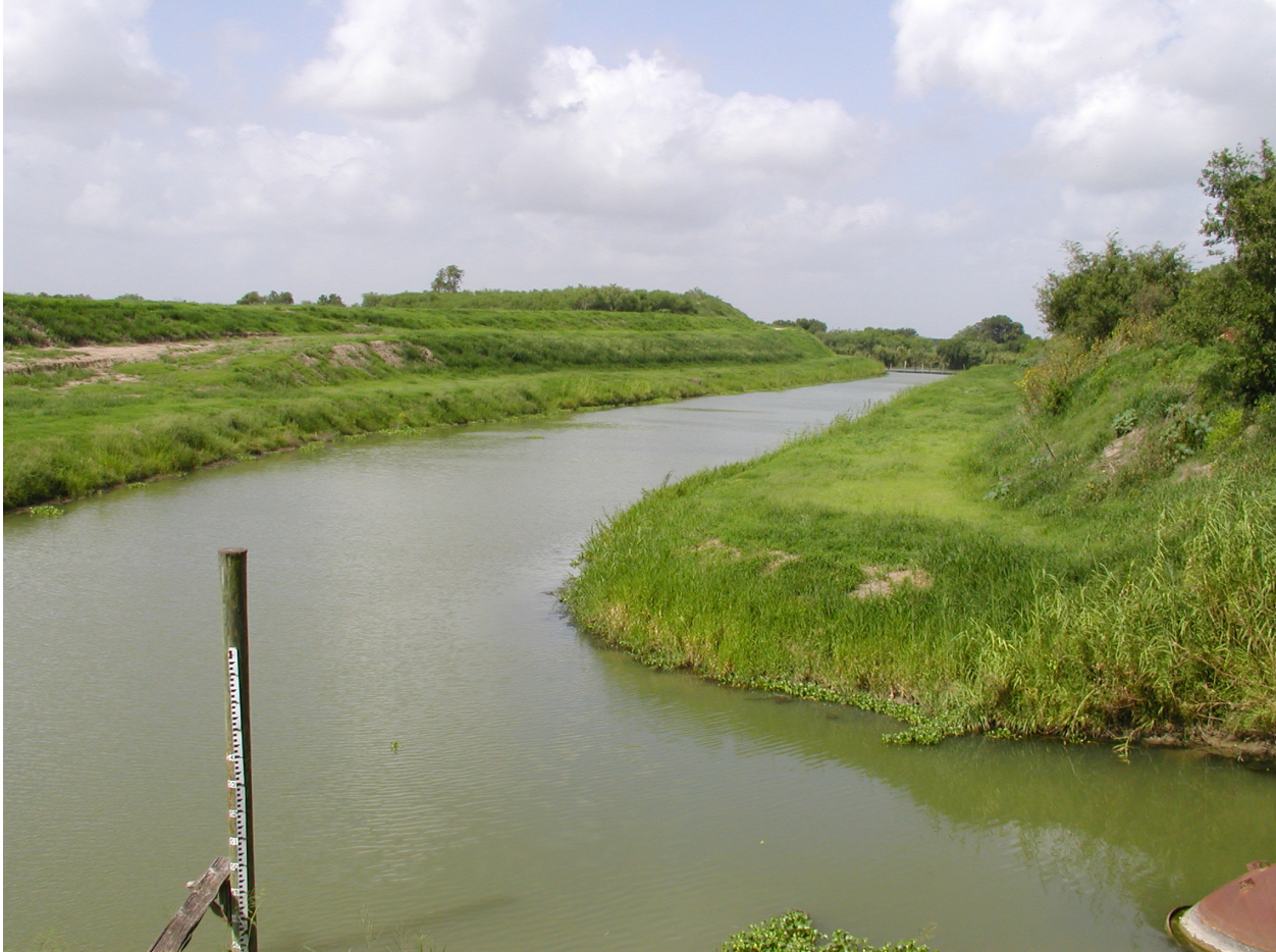
EXHIBIT C1. Constructed Inlet Canal System off the Rio Grande Leading to Harlingen Irrigation District Cameron County No. 1's Pumping Plant, 2003 (Wolfe).
