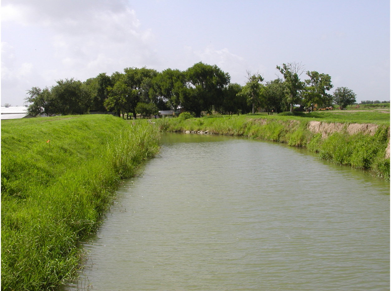
EXHIBIT C4. Harlingen Irrigation District Cameron County No. 1's Main Canal, 2003 (Wolfe).
