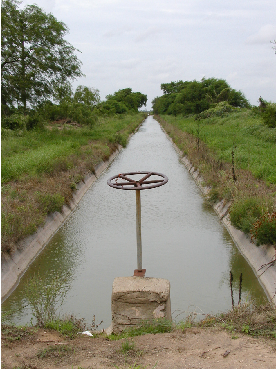
EXHIBIT C6. Harlingen Irrigation District Cameron County No. 1's Concrete-Lined Canal With Gate, 2003 (Wolfe).
