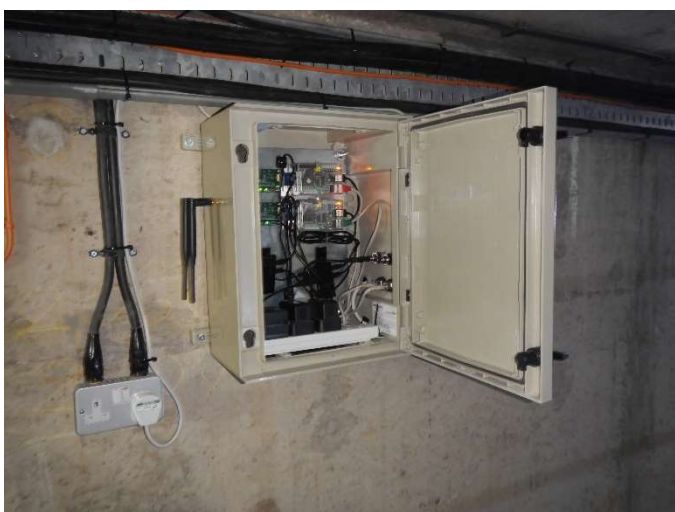
Figure 4. New gateway installed in 2013. Photo: Authors. (Photograph taken November 2017)
