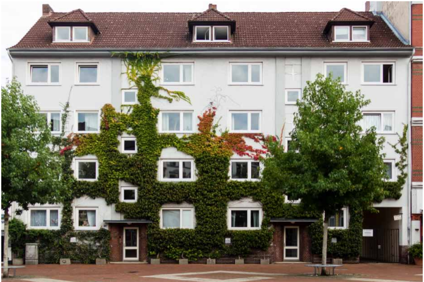
Fig. 13 - Green facade. Hamburg, Germany. 2016. Photo by D. Huntington
