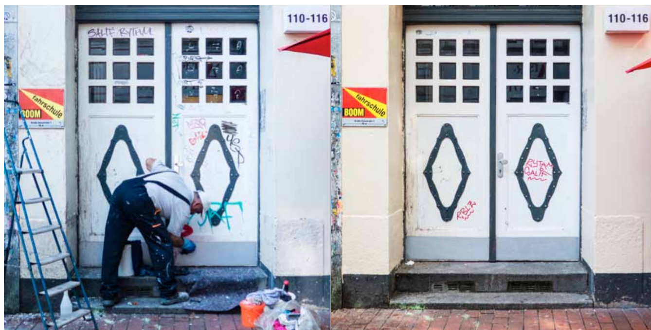
Fig. 2 - Left: Chemical-based graffiti management efforts on 5 September 2016. Right: New graffiti tags appear on 17 September 2016. Hamburg, Germany. Photos by D. Huntington.
