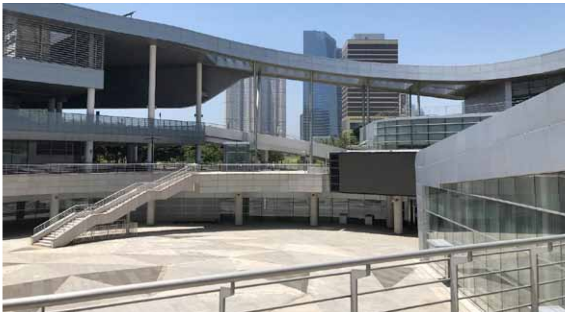
Fig. 1: Songdo in the metropolitan area of Seoul in South Korea is another famous example for a smart neoliberal city project that failed, because nobody wants to live there. Even though it is nearly empty, construction on high-rise buildings still goes on, in hope of future developments.
