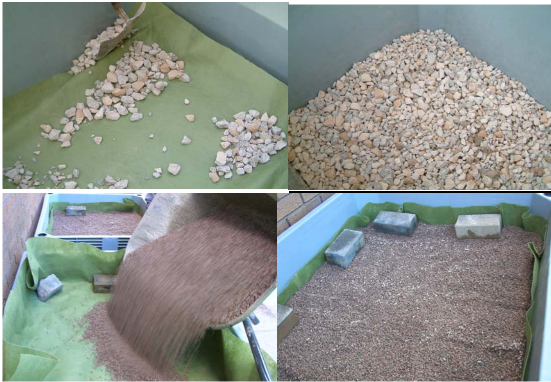
Figure 7.1 Showing Construction of the PPS Model for Out-door Infiltration Experiments
