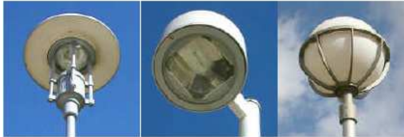
Figure 13: A New Campus Light Fixture, A Parking Light, and a Discontinued Campus Light Fixture
